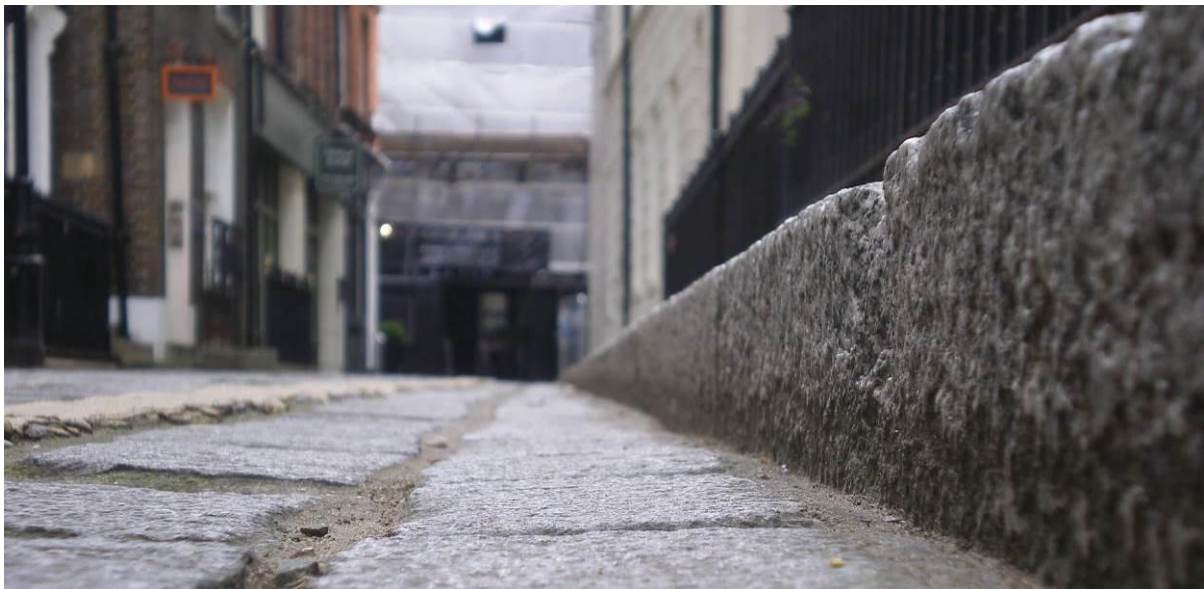
Took's Court, kerb detail
